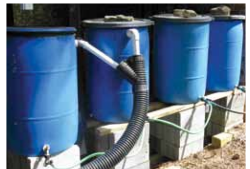
Daisy chained rain barrels with Y-connectors.
