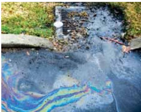
Stormwater entering a storm drain, leading to waterway untreated.
