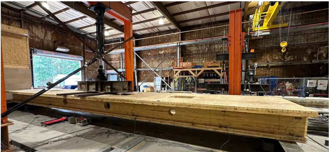
Construction of the first of two, 40' span, mass timber systems tested in the summer of 2024 at the Built Environment Lab
