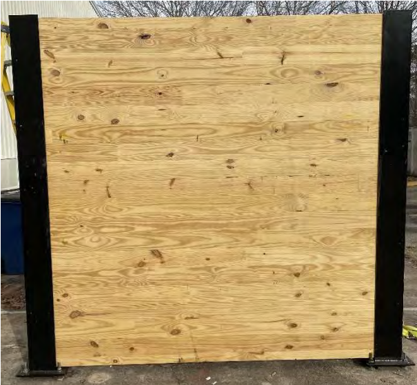
Construction of the second CLT noise barrier in December 2023 (left) and currently (right) with no coating
