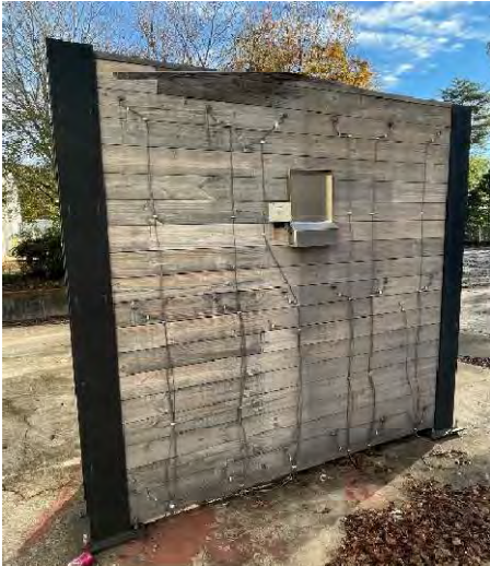
Construction of the first CLT noise barrier in August 2021 (left) and currently (right) with two UV coatings
