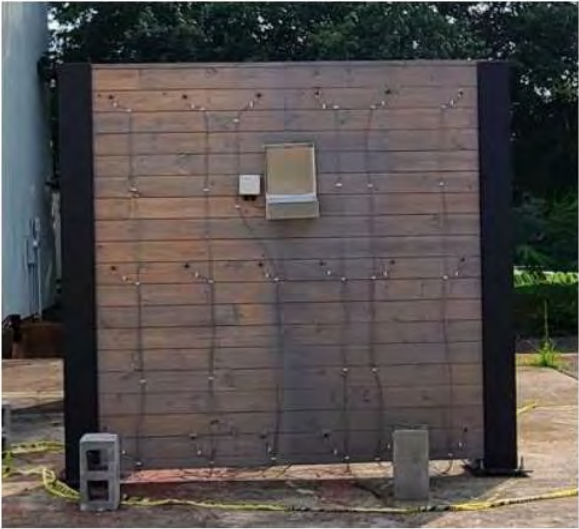
Construction of the first CLT noise barrier in August 2021 (left) and currently (right) with two UV coatings
