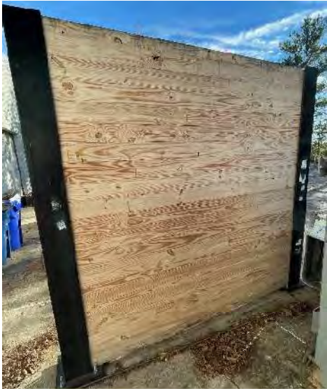
Construction of the second CLT noise barrier in December 2023 (left) and currently (right) with no coating
